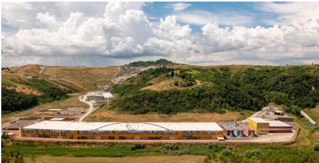
Figure 8: The anaerobic digestion plant inaugurated in 2024. Source: Belvedere SpA, website
